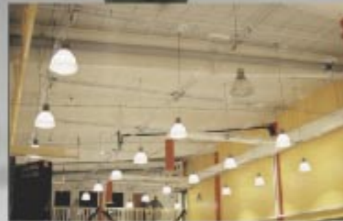
In this application 2,5 metre support distance - a substantial installation cost reduction!
