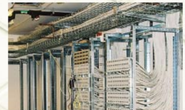
CombiRack - use Full access - full control. Racking and cable channelling in one robust system.
